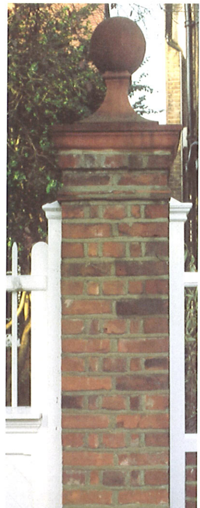
Brick pillar topped with ball finial
