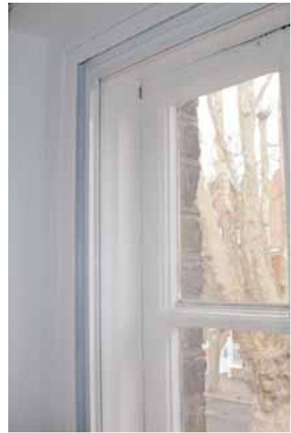
Horizontal sliding secondary glazing applied to a French door
