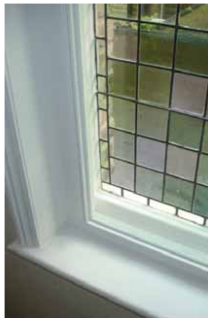
“Lift-out” secondary glazing applied to a fixed stained glass light
